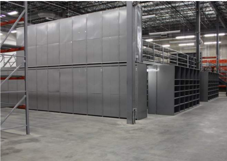
Shelving Supported Mezzanine
