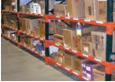
Structural steel rack
